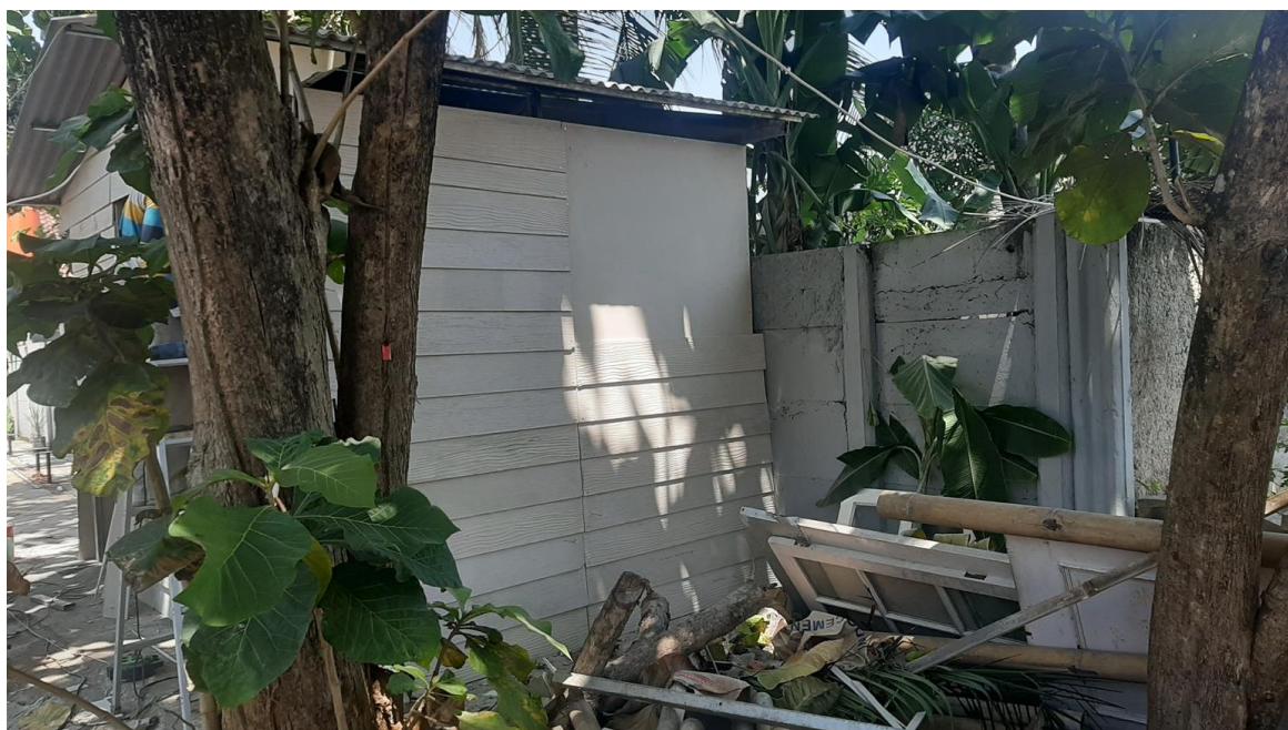
Figure 4. Installation of Patterned Concrete Panels on The Right Side
