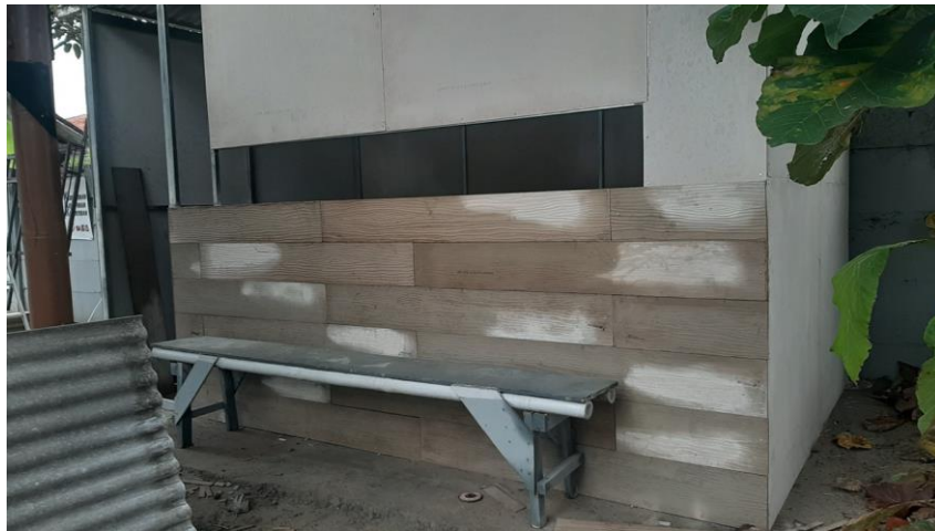
Figure 1. Plain Concrete Panel Installation
