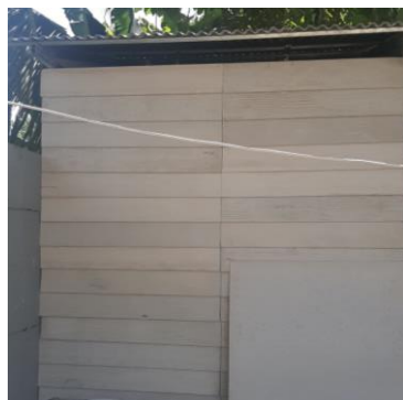
Figure 2. Installation of The Left Side Patterned Concrete Panel
