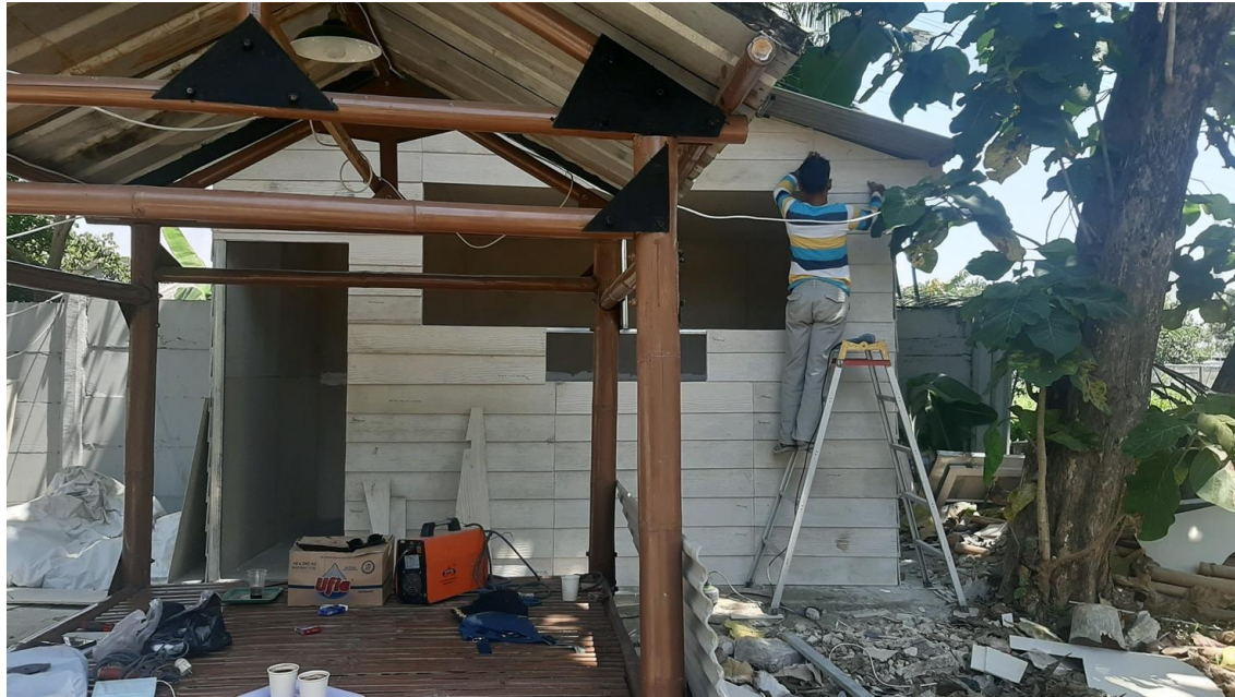
Figure 3. Installation of The Front Side Patterned Concrete Panels
