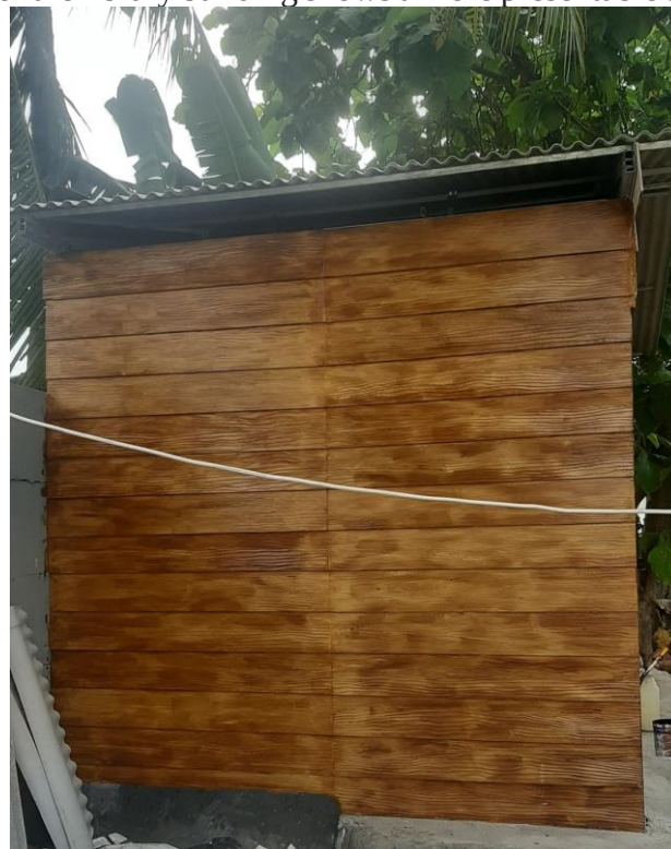
Figure 6. Left Side Patterned Concrete Panel Coloring
