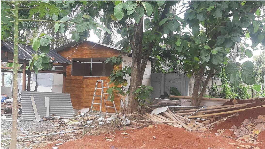
Figure 5. Front Side Patterned Concrete Panels Coloring
