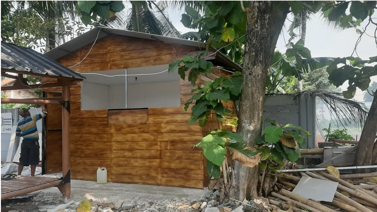
Figure 7. Finishing of Concrete Panel
